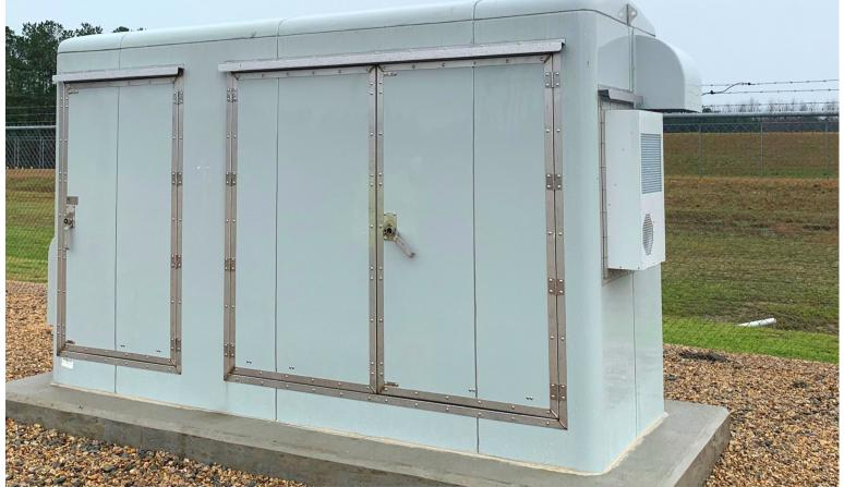
Insulated and air-conditioned enclosure reduces battery overheating and ensures longer battery life.
