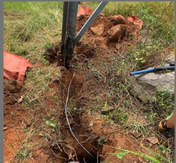
Cathodic Protection Anode Installation on Grillage
