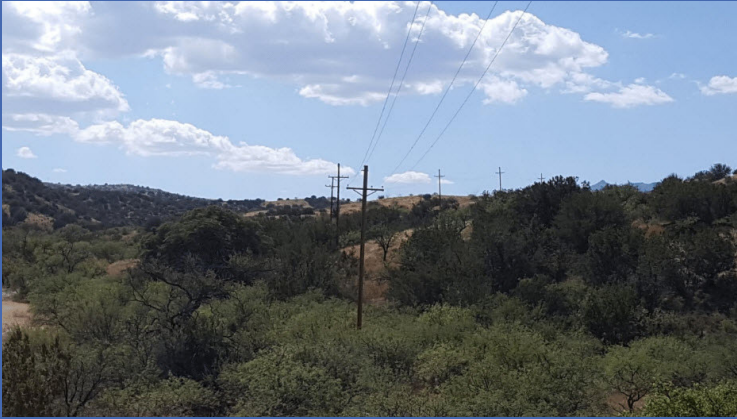
Rough Terrain Inspection
