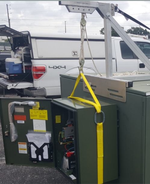
Lifting device developed to aid in installation.
